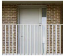
House entrance door - Solid flush external entrance door with glazed sidelight
